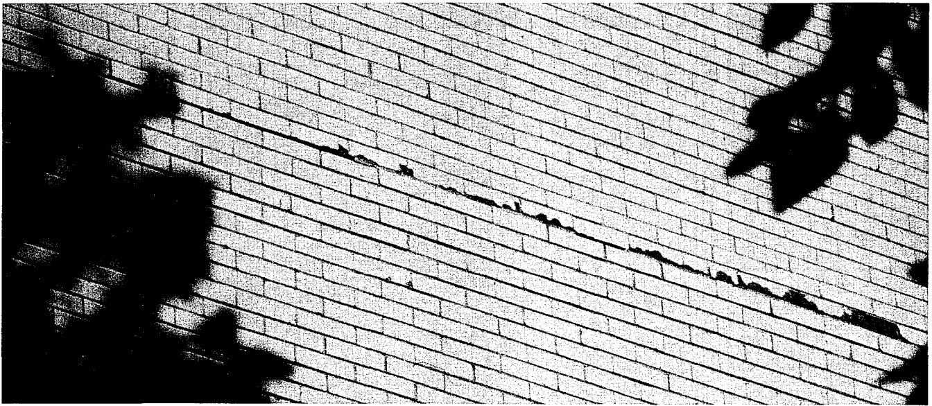
FIG. 2. Spalling of masonry veneer at a steel shelf angle location.
